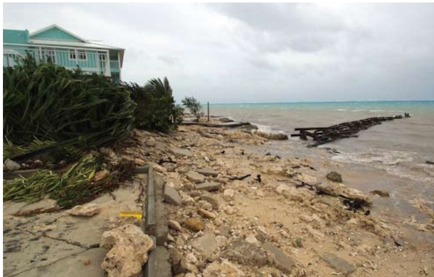
The remnants of a dock destroyed by a hurricane.
